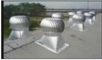
Gambar 10. Turbin Ventilator
